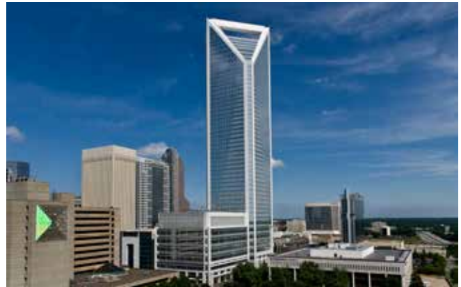
Duke Energy Center, Charlotte, North Carolina
