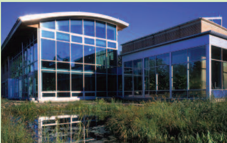
The Adam Joseph Lewis Center for Environmental Studies at Oberlin College is a 13,600 sq. ft. all-electric building that produces at least as much energy as it uses in a year through a roof-mounted 60 kW photovoltaic (PV) system and a 100 kW PV system located over the parking lot.
