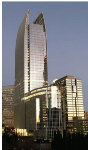
1180 Peachtree, managed by Hines, uses captured and stored storm water and condensate from the building's mechanical system.
